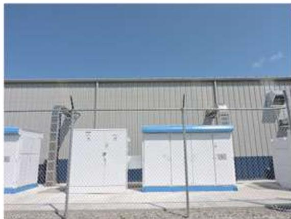
Figure 5: Power Busway Eaton 2MW Inverters &amp; Transformer
